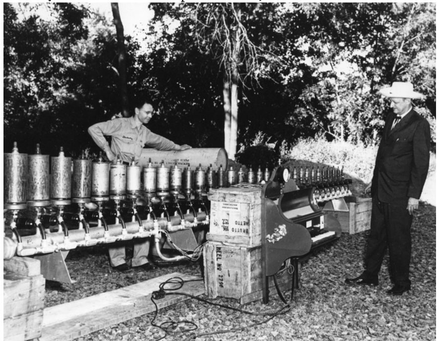
E. J. Quinby inspects the new manifold and electronics. Man on left unknown. Photo courtesy PLCHC Inland Rivers Library.
