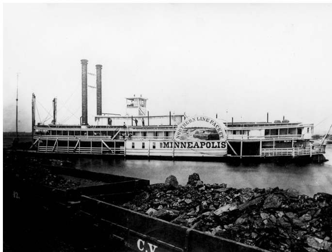
MINNEAPOLIS (3944) . Like DUBUQUE , her hull was built in Wheeling and then taken to Pittsburgh for completion in 1869. Engines 30's with 7-ft. stroke. She measured 233 x 36 x 5.8. In May 1882, Sam Clemens took passage from St. Louis to Hannibal on GEM CITY , then transferred to MINNEAPOLIS for remainder of trip to St. Paul. He was gathering material for his new book Life on the Mississippi .
