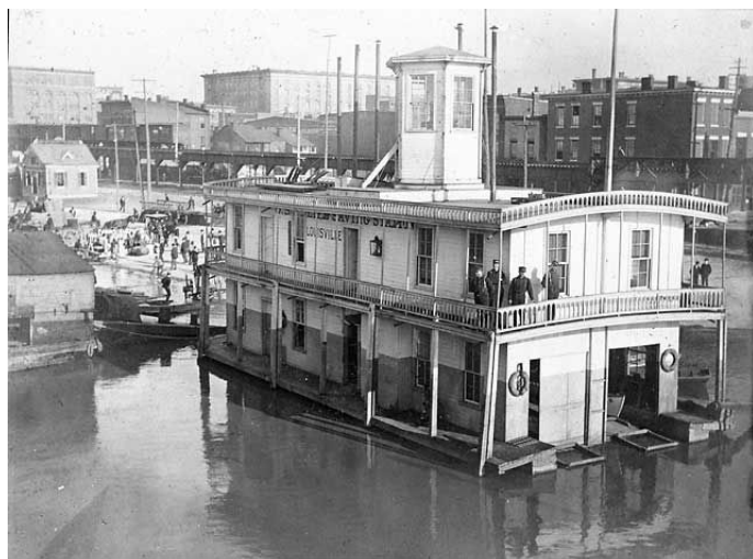
View of station showing the opening in lower end through which lifeboats were launched and retrieved from the river.
