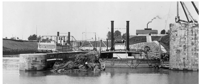
U. S. Engineer's MAJOR MACKENZIE (on left) attempted to prevent ice and drift from blocking the canal in January 1895. The ice wrecked her wheel and sank her three barges.
