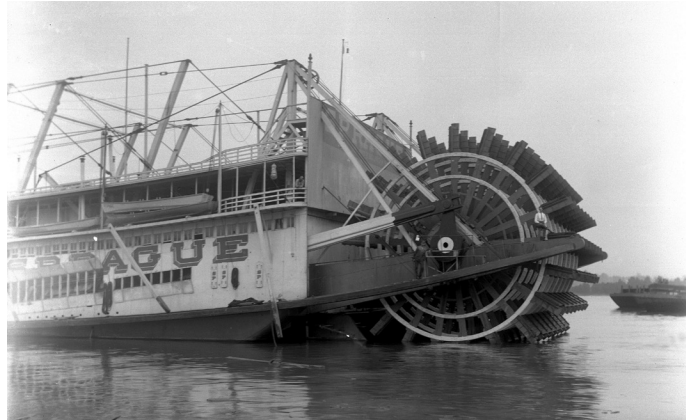
Big Mama waits for installation of two pumps at Howards.
