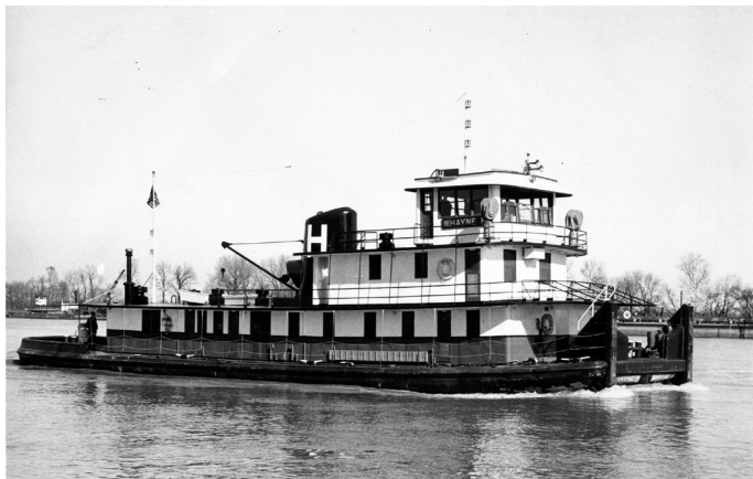
WHAYNE H. , second boat of that name. Built 1948 as ALEX SMITH , twin props, 111 x 26.5 for Charles C. Smith Co. of Houston, who sold her soon after completion to Houglan Barge Line of Paducah. Photo courtesy of Boat Photo Museum.
