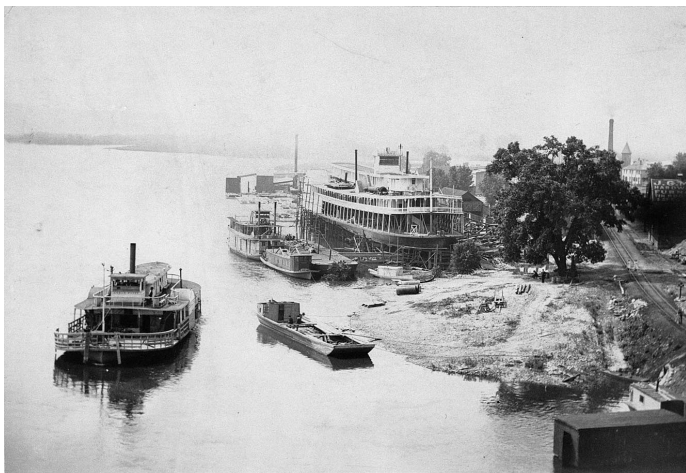
SAINT PAUL high and dry for rebuilding at the Eagle Point marineways in Dubuque. The ferryboat EAGLE POINT appears on the right. This most likely was taken in 1903 from a span of the Eagle Point highway bridge which opened the year before. From Murphy Library, Univ. of Wisconsin-LaCrosse.
