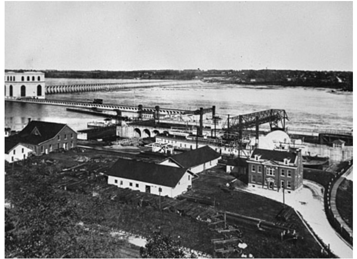
RR transfer ALBATROSS being lengthened in drydock, 1920. 13 years earlier she would not fit through the locks; now this was the only inland drydock large enough to accommodate her.
