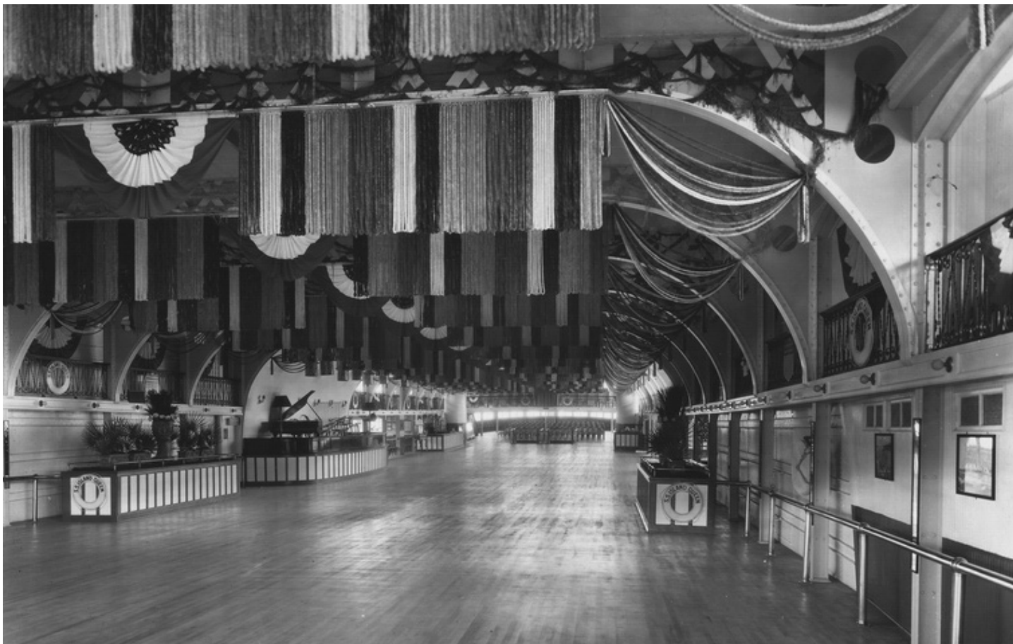
Pictured above is the ballroom deck looking forward. In the far center of the photo you can see the two stack jackets which carried the smoke and fumes from the boiler breaching up through the stacks above. Her bandstand is on the port side about midship, within easy earshot of either end of the dance floor. The view below is looking toward the stern. These photos were taken March 31, 1929. Both the ISLAND QUEEN and PRESIDENT featured the balcony or mezzanine overlooking the dance floor from the deck above.
