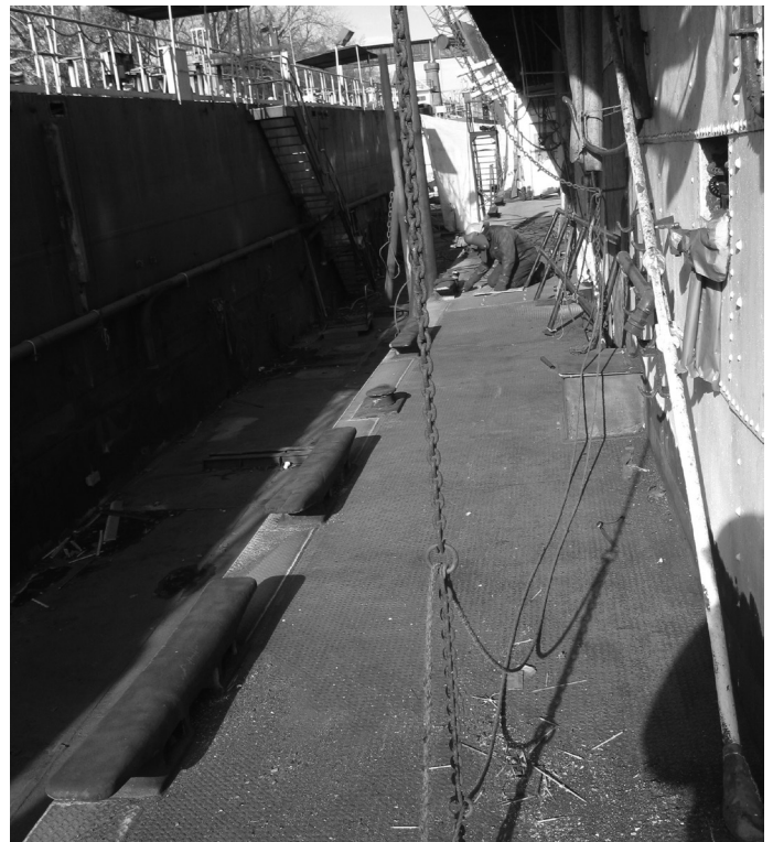
Workman replacing some of the main deck plating.
