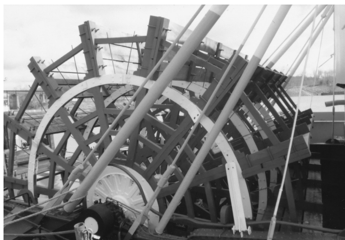
Completed wheel painted and ready to roll. Buckets were left unpainted.
