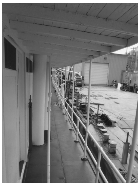
Boiler deck guards outside cabins with original red tile paint, formerly "red lead," same as wheel and main deck.
