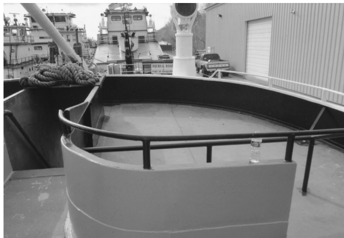
Coal bunker area with new deck plate installed.
