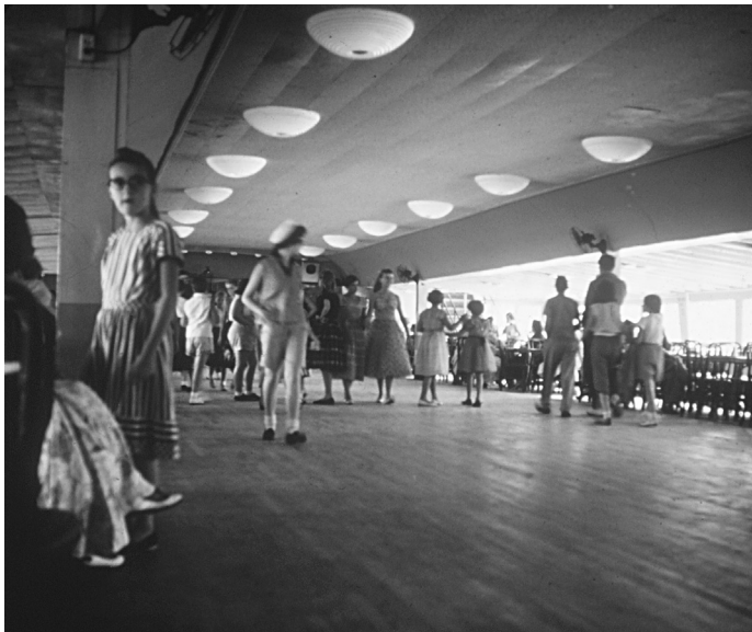
The boat's 33 by 96-foot maple dance floor looking toward stern. By this time, the pressed tin ceiling had been replaced with more modern acoustical tile.
