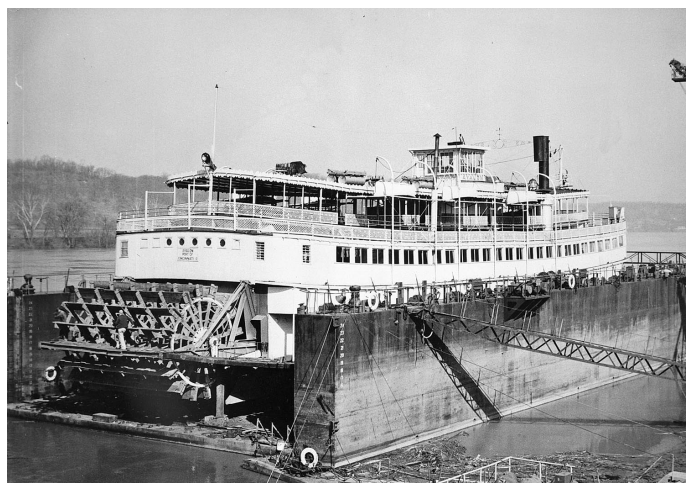
On drydock at Marietta Manufacturing Co. in Point Pleasant, WV, spring 1955 for addition of sponsons to her hull. Both photos from editor's collection.
