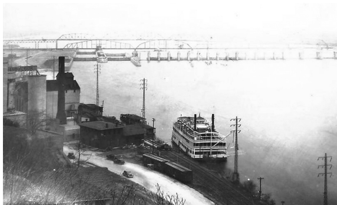
IDLEWILD at her Alton, IL landing some time after Lock & Dam 26 was completed in mid-30s. The new Clark Highway Bridge in distance opened months before IDLEWILD arrived at St. Louis. Both photos this page courtesy Murphy Library.
