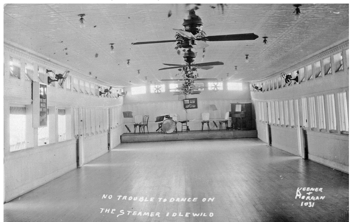
The steamer's 33 by 96-foot maple dance floor was enclosed by side bulkheads with windows and skylight transoms. Photo courtesy of Murphy Library, Univ. of Wisconsin - LaCrosse
