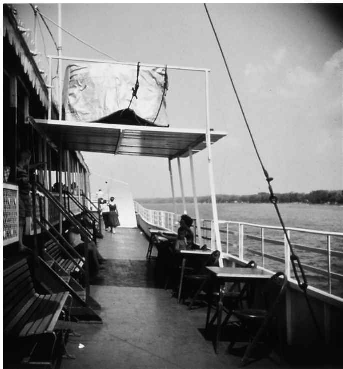
Above: Hurricane roof and texas looking forward on port side in 1957. Below: Three years later, the old wire mesh railing around the edge of the hurricane roof had been replaced with sturdier steel bulwarks in this same location looking aft.
