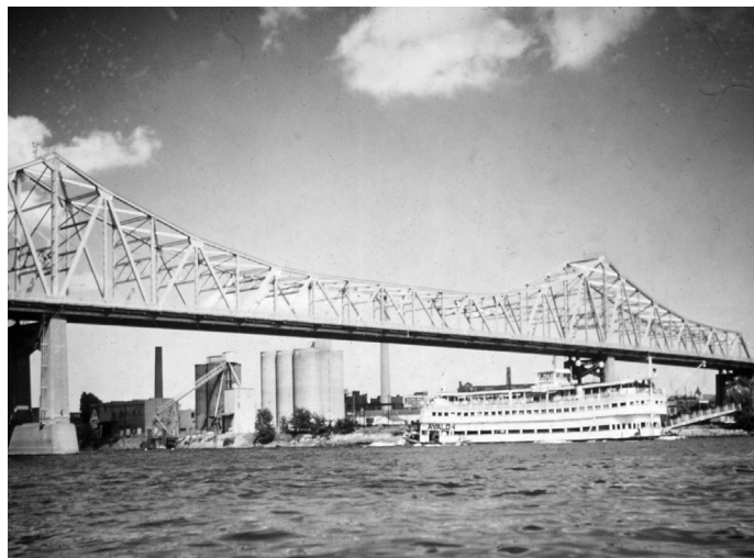
Under the Cass Street Bridge at La Crosse, WI.
