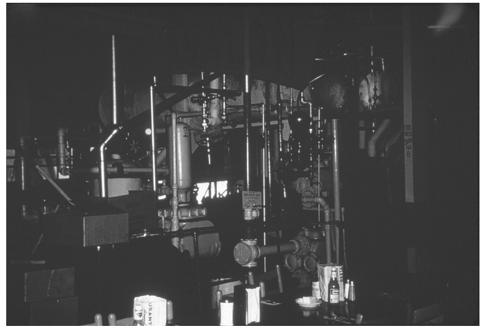
Deckroom with dining tables for officers and crew located just aft of cookhouse, boilers and pumps.
