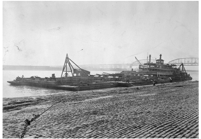
Another dramatic photo of the boat at St. Louis with her tow of construction equipment for building Lock and Dam 22 at Saverton, MO in February 1934. Murphy Library photo.
