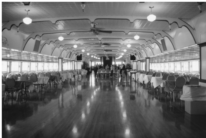
BELLE's elegant, renovated ballroom with refurbished woodwork and restored original-style pressed tin ceiling.
