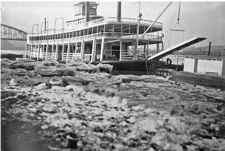
The steamer is completed except for outfitting in this view taken in late December or early January 1915. Her departure was delayed by ice, visible in the foreground. Two workmen appear on a barge or flat off her port bow, while a ladder is still propped alongside her mast.
