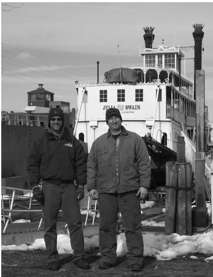
Capt. Carl Henry (L) and Capt. Eric Dykman pose on a cold, blustery February 11th afternoon while work progresses on JBS
