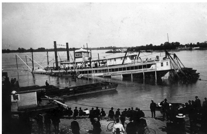
GEORGIA LEE, pictured on our front cover, appears in this unfortunate view in May 1909 at Paducah Marine Ways. She was being hauled out for repairs when the marineway chains gave way and she took a run for the river and sank offshore. Photo courtesy of James Lee Sr.
