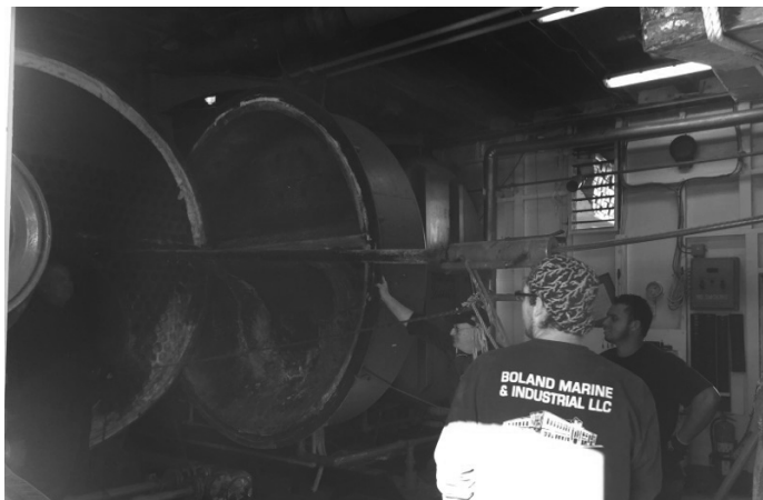
Above: Pulling tubes out of boiler, a laborious process. Below: Captain's Salon stripped bare of its furnishings.
