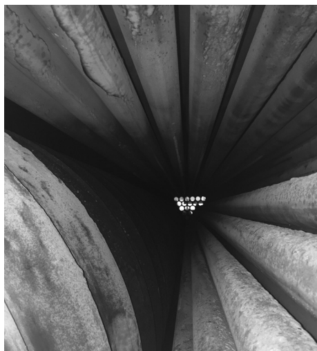
Right: Matt's pet project: painting the manifold and polishing calliope whistles. Below (L to R): Removing old emergency generator; A rare look inside the NATCHEZ boiler. Old tubes have been removed and boiler prepped for the installation of the new tubes; Dance floor after stripping and revarnishing.
