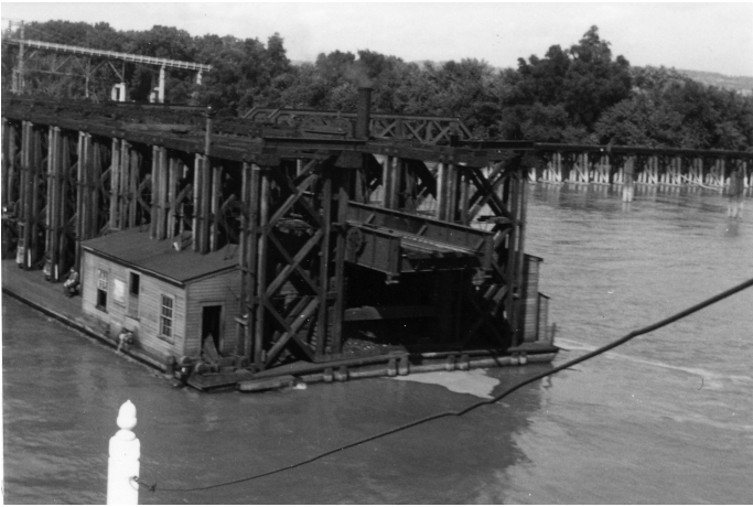
Top: Main cabin of GORDON set up for dinner. Middle: Shore stop above McGregor to board two members of Bickel family. Bottom: Floating pontoon railroad bridge at Marquette. There was a similar one at Reads Landing in previous times.
