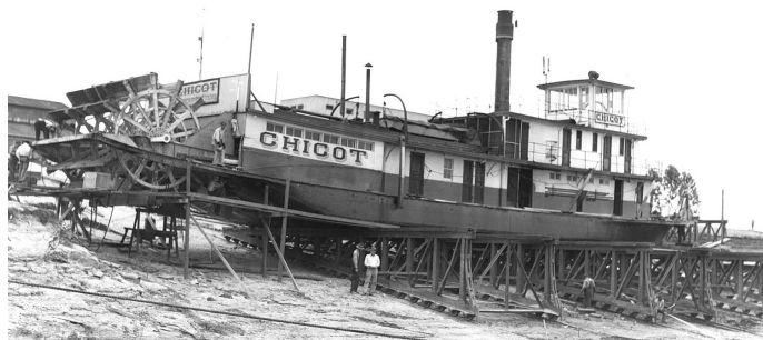
CHICOT (To413) built 1925 by Howards for USE Vicksburg District. G&E engines 10's - 5 foot stroke. Sold 1941 to Commercial Barge Lines of Evansville. Murphy Library photo
