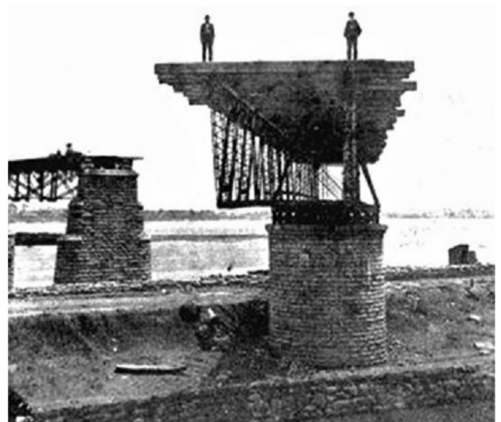
Swing span of Ohio Falls Bridge at entrance to Canal under construction in 1870. Courtesy of historiclouisville.weebly.com
