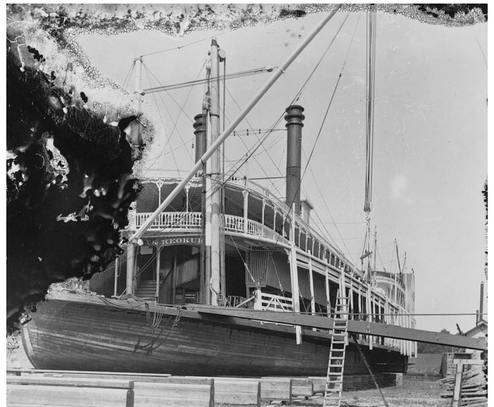
1896 view of QUINCY under renovation on Diamond Jo ways at Eagle Point, five years after her acquisition and rebuilding from Davidson Line's GEM CITY. Murphy Library photo.
