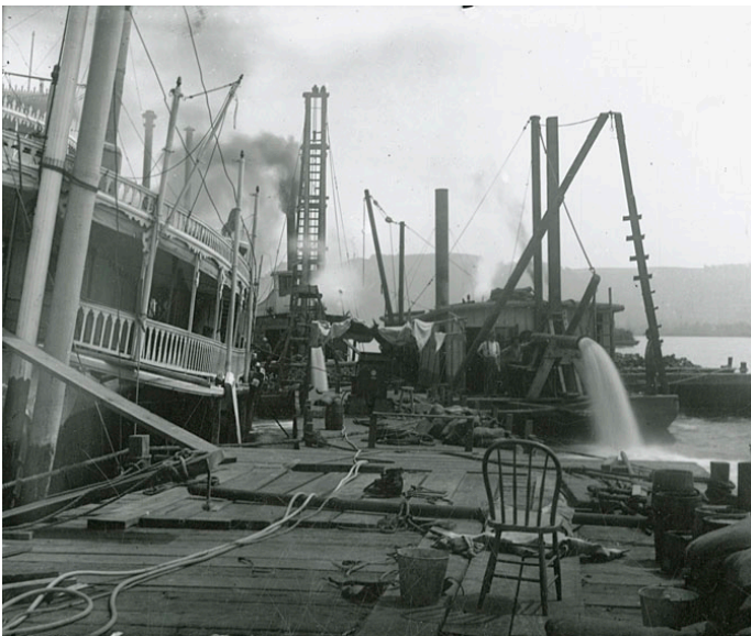
Capt. Killeen's salvage and boatyard crew pumping out the hull of QUINCY after temporary patches were in place. Photo from Murphy Library, Univ. of Wisconsin - La Crosse
