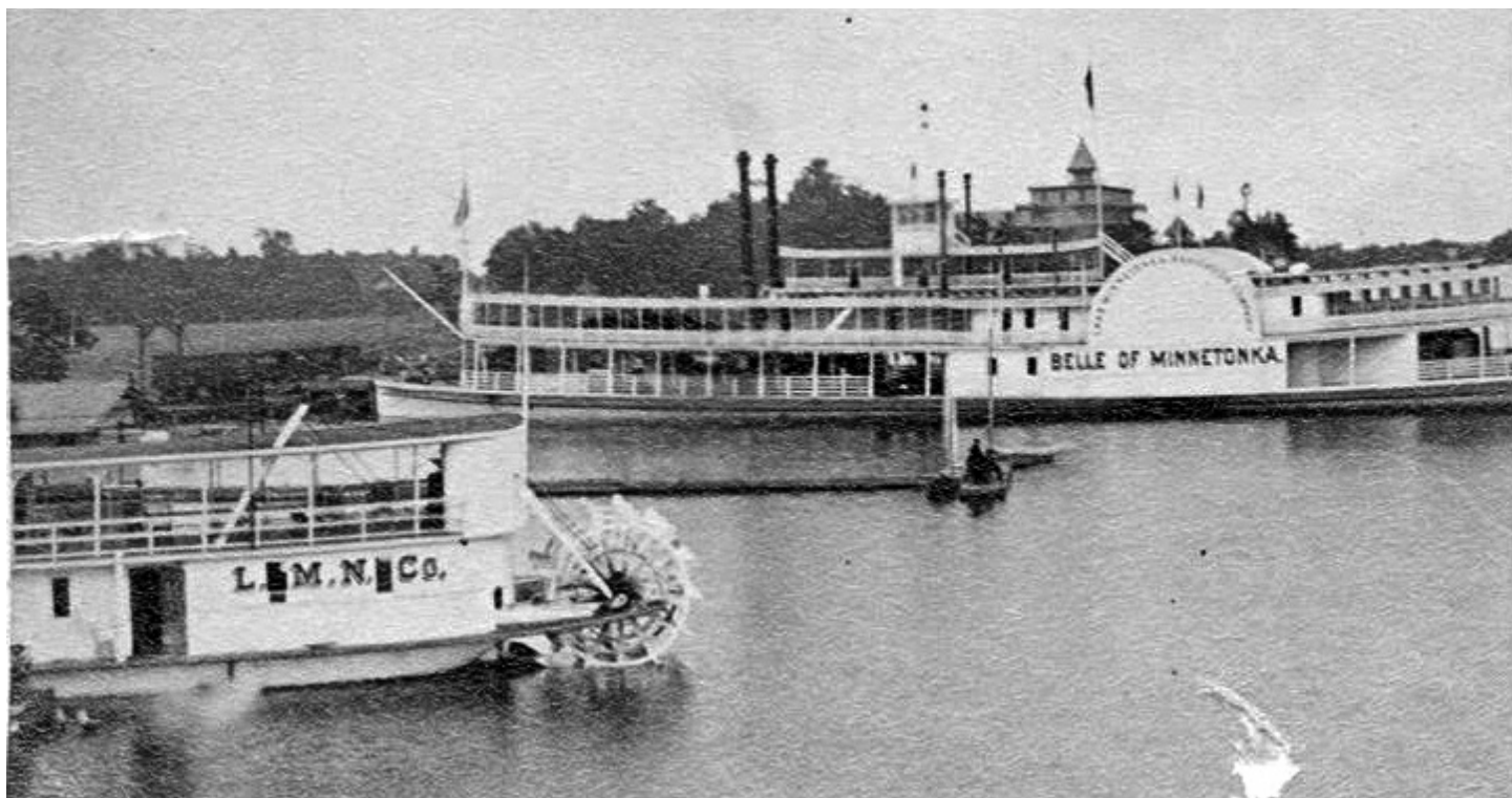
Capt. Peyton S. Davidson supervised building of BELLE OF MINNETONKA on a hull 288 x 60. Her engines, from the famous PHIL SHERIDAN were 22's - 7. Photo taken at Wayzata with Arlington Hotel in background. Launched on July 4, 1882. On July 5th, the wind caught her and drove her into pilings, knocking a hole just above the waterline. Her passenger capacity was later upped to 2500, but she proved too large to be operated economically on the Lake. Photo: Excelsior-Lake Minnetonka Historical Society.
