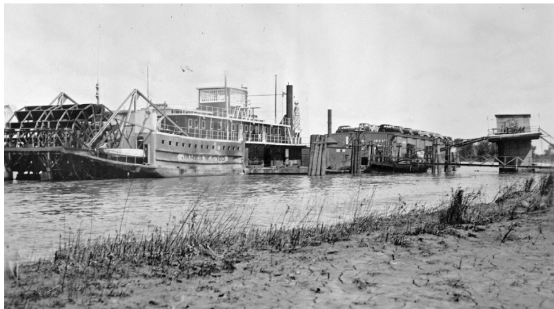
Above: Str. JAMES W. GOOD (T1340) with auto barge for delivery below St. Louis from Ford's Twin Cities Assembly Plant. Below: FBL "express Barge" MOBILE (T1844), 280.1 x 49.1 x 10 was a self-propelled freight barge, shown here carrying Fords in 1932. Murphy Library photos.
