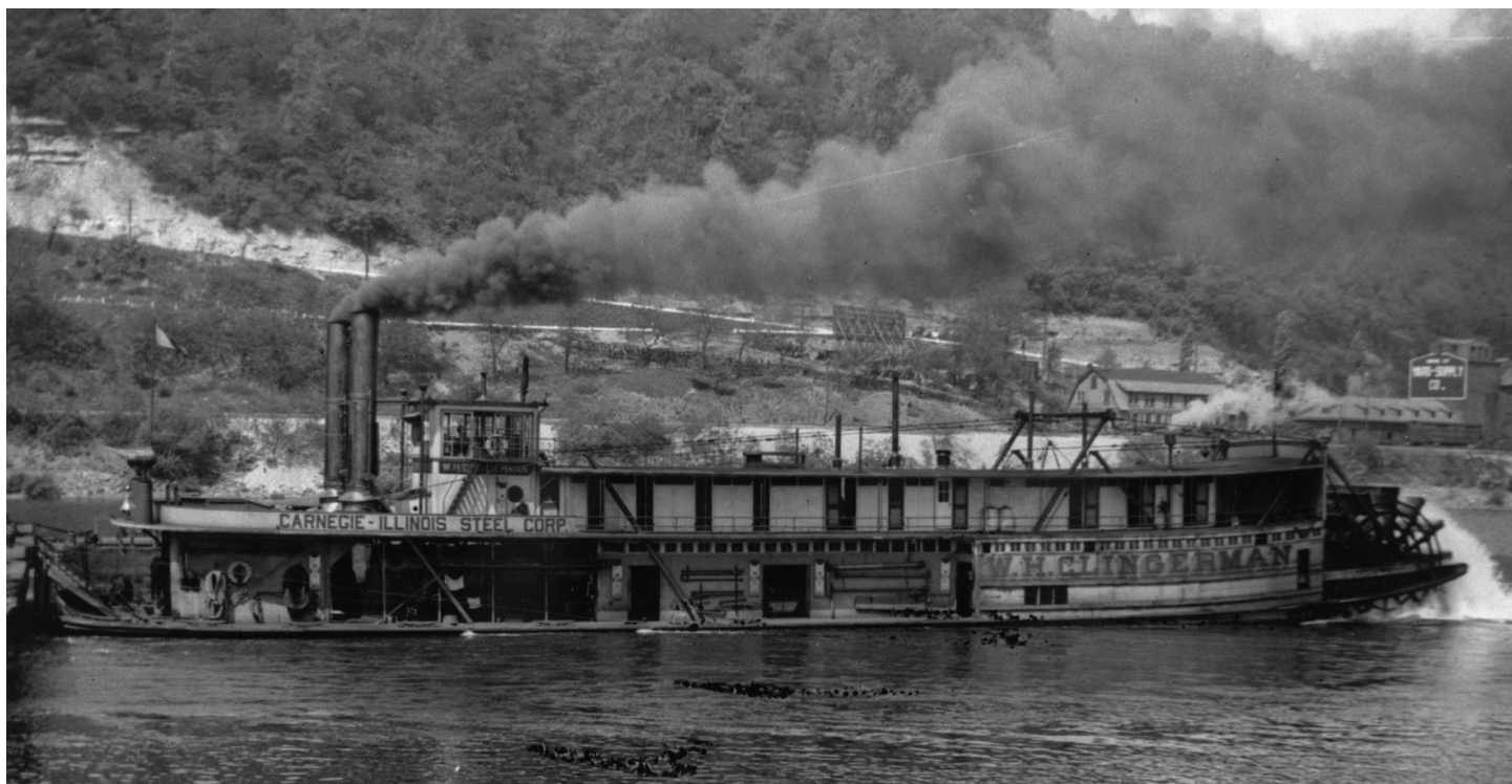
SNYDER in her early years as W. H. CLINGERMAN. Her hull was widened by 4 feet in 1930 to increase stability. Since the James Rees and Sons boatyard closed that year, it is uncertain whether the work was done there. Photo courtesy of Murphy Library.
